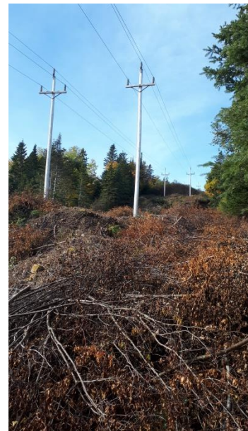
The trail follows the transmission line here. Consider some re-routes.
